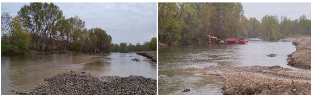
Figure 2. Addition of gravel and pebbles to the riverbed to improve connectivity with the secondary channel
