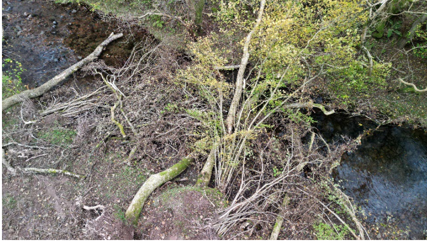
Fig. 3: Area view of large wood accumulation achieved through winching and chainsaw felling
