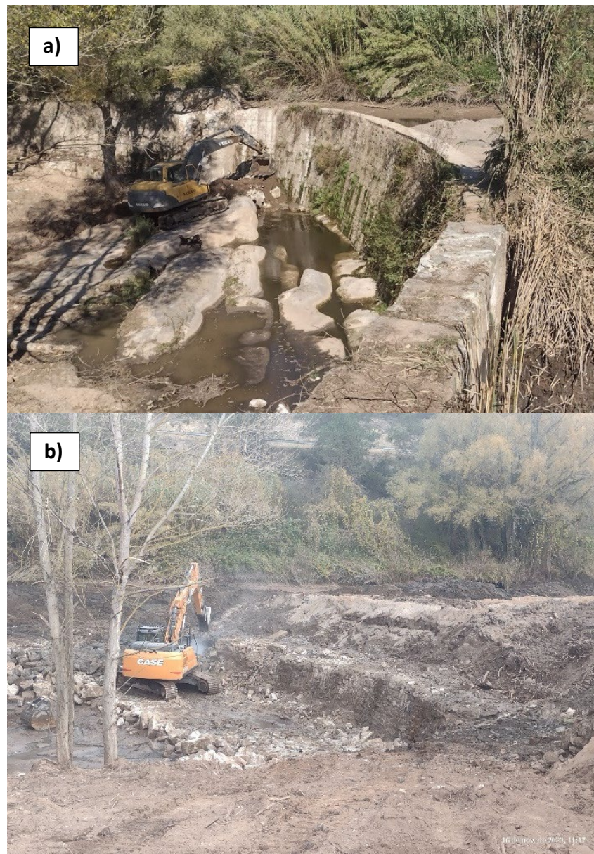
Figure 1.- View of the Colonia Rio dam before (a) and after (b) the demolition of the barrier.
